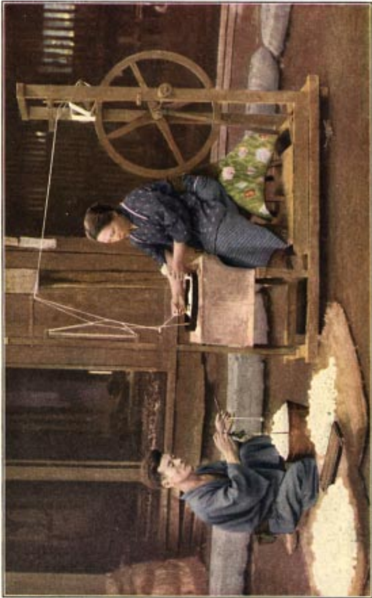
REELING THE SILK FROM CORTICELLI COCOONS BY FOOT POWER, CALLED "RE-REEL" SILK.
